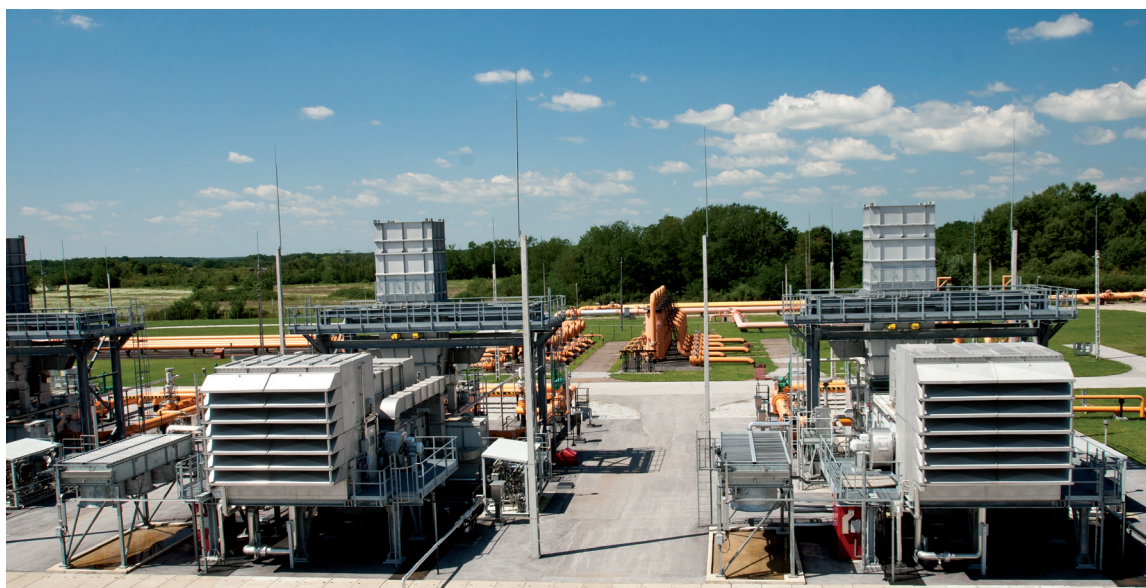
Beregdaróc compressor station
