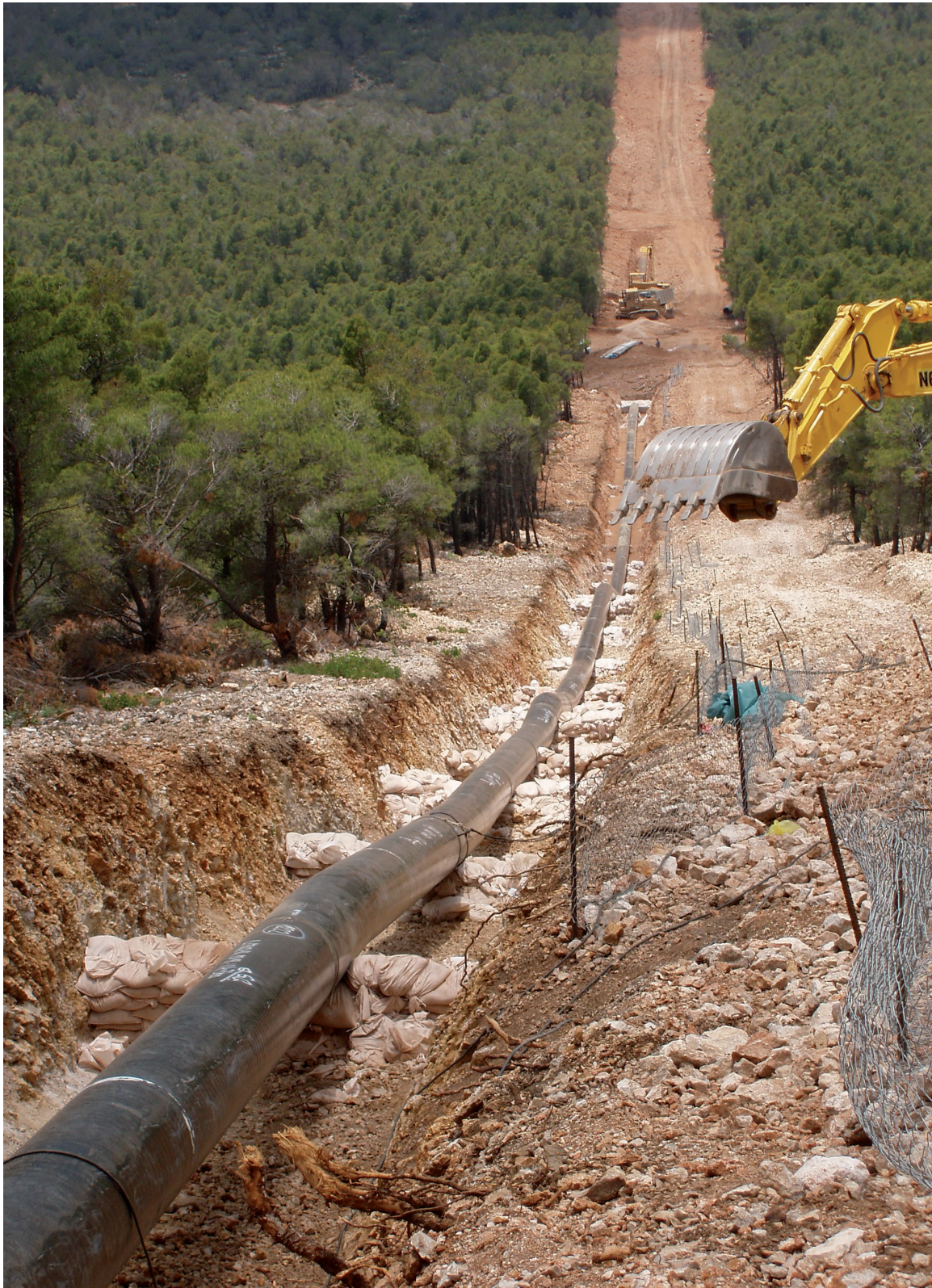
Steep slope pipeline construction in Corinth branch
